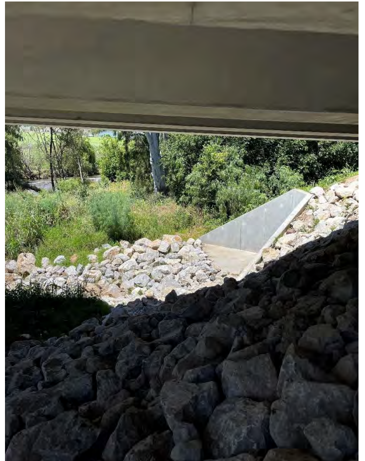
Figure 4 Headwall underneath the highway bridge
