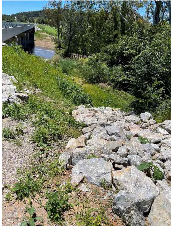
Figure 1 Rock lined outlet to Namoi River
