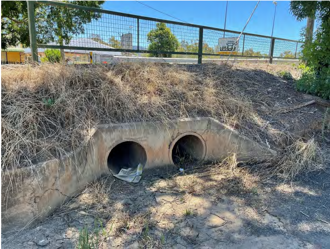
Figure 12 Culvert underneath old bridge
