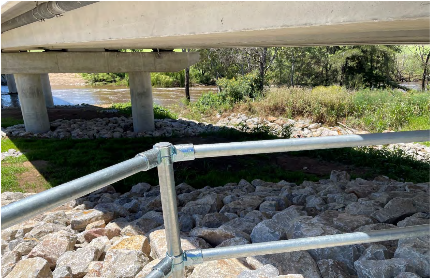
Figure 5 Headwall underneath the Highway bridge
