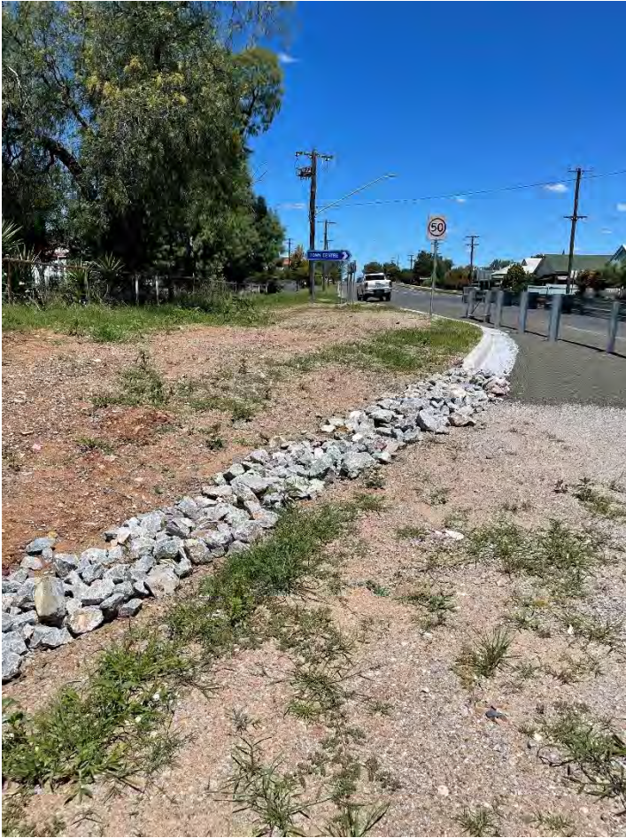
Figure 2 Manilla St kerb outlet to Namoi River near the new highway
