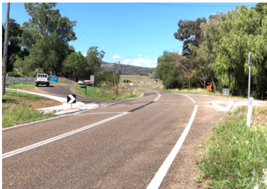
Photo of pedestrian safety improvements at Dungowan Primary School
