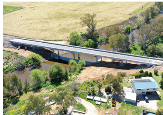
Photo of new Manilla Bridge over the Namoi River
