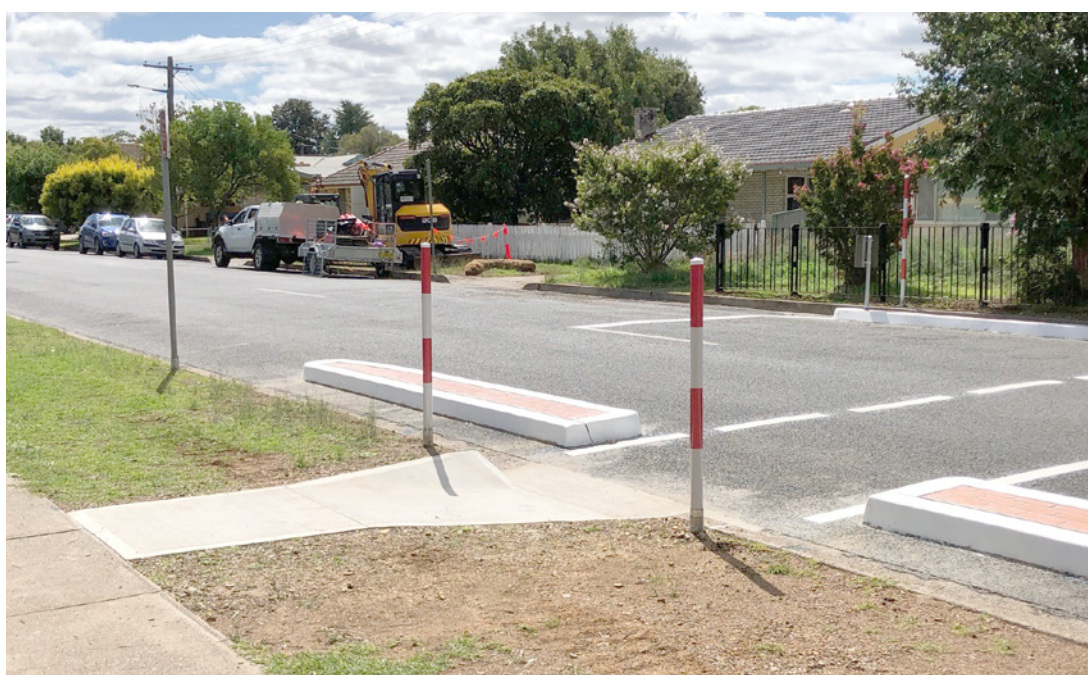
Photo of crossing outside of South Tamworth Primary School
